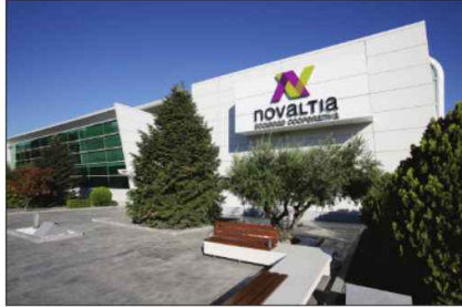
Novaltia's distribution centre in Zaragoza, Spain.
