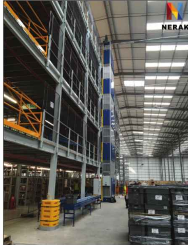
One of two lifts supplied by Nerak to Missguided's new warehouse in Trafford Park, Manchester.
