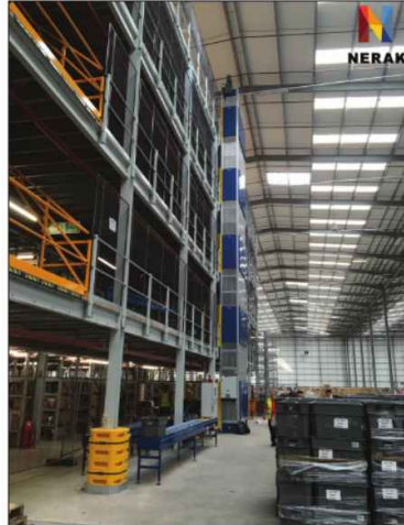
One of two lifts supplied by Nerak to Missguided's new warehouse in Trafford Park, Manchester.
