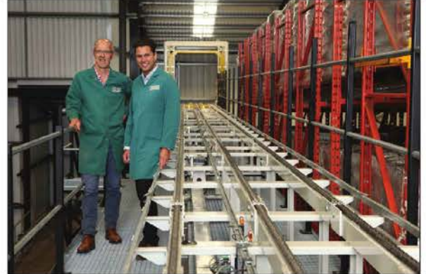
Left to Right: George Page (Production Director) and David Wilson (Operations Manager) with the new central conveying system.
